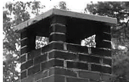
Concrete Cap Chimney Top
